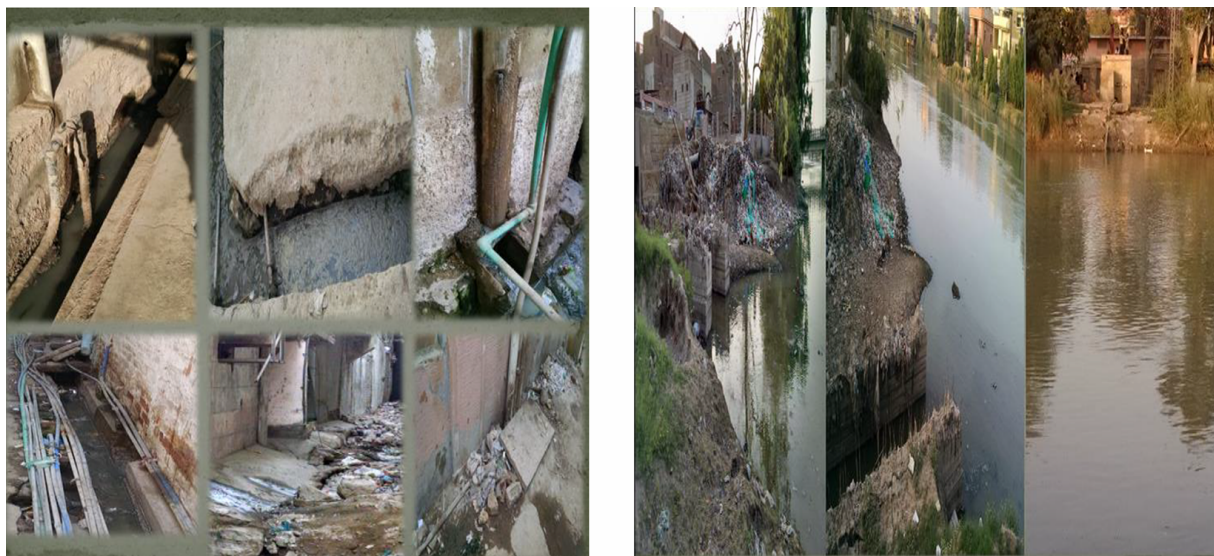
Figure 2. Water supply pipes laid parallel to sewerage drains (Right); excreta discharges into the canal and supply pipe (left)
